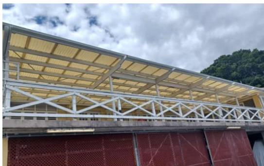
New guttering installed on the deck. No more dripping!
